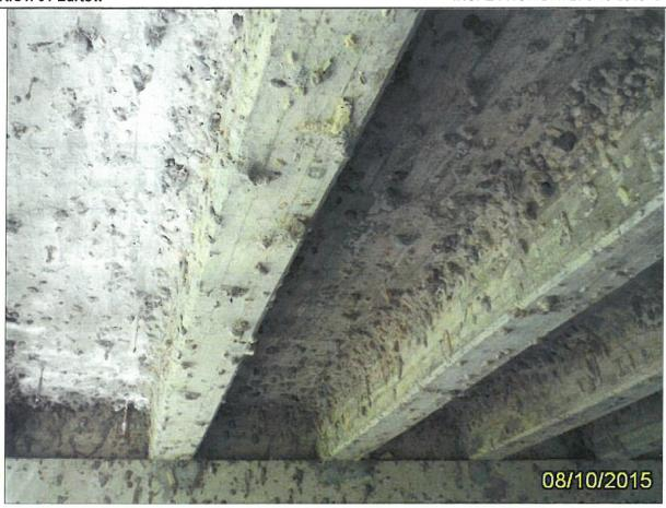
Photo 1 - Elements 13 Unp Conc Deck/AC Ovl & 110 R/Conc Open Girder
