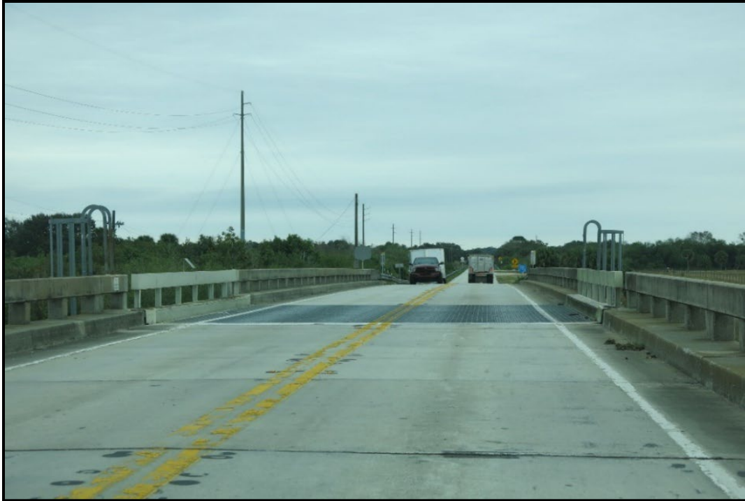
Photo 1. SR 70 over Kissimmee River Bridge, Bridge No. 910001 (8HG01236/8OB00336), looking east. Note the removable steel span.
