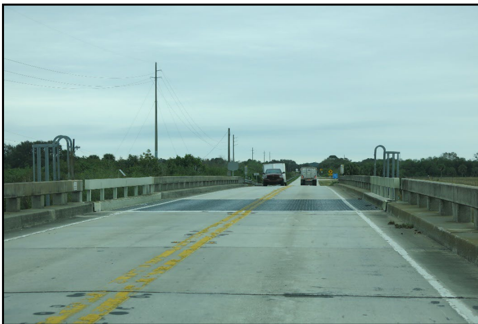
Photo 5.2. SR 70 over Kissimmee River Bridge (FDOT 910001) (8HG01236/8OB00336), looking east. Note the removable steel span.
