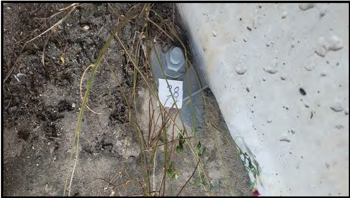
Photograph 40 View of Asbestos Homogeneous Area 13 – Rubber – Vibration Pads of Bridge 910001 (Sample Location 38).
