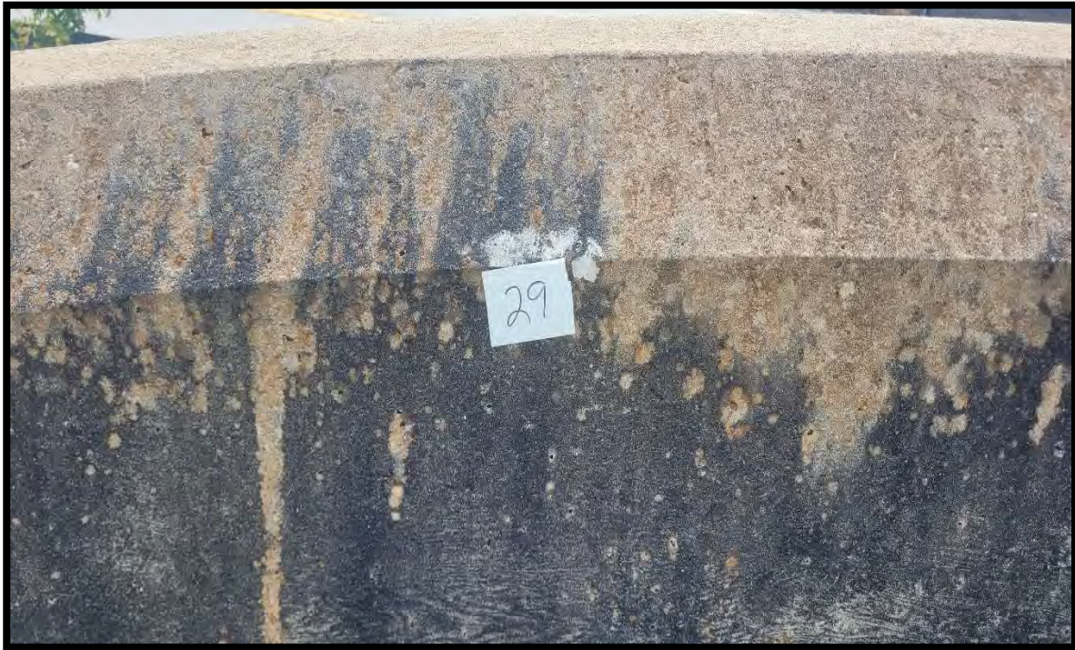
Photograph 31 View of Asbestos Homogeneous Area 10 – Concrete, Class V Coating – Landside Buttress of Bridge 910001 (Sample Location 29).
