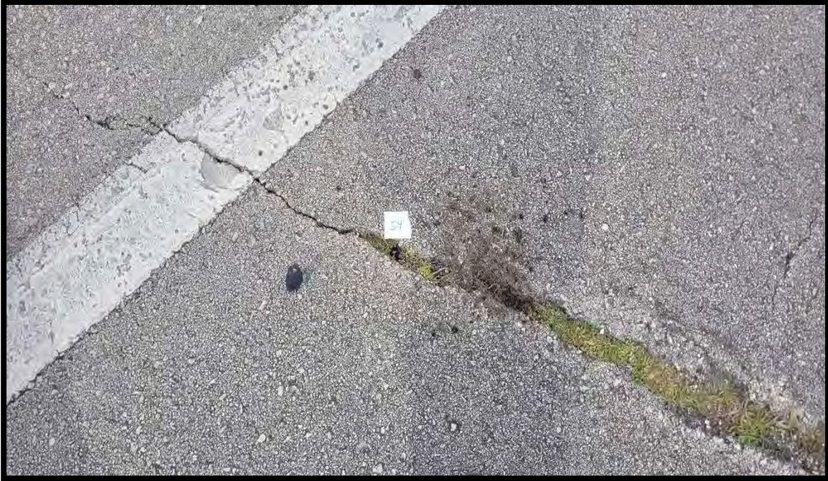
Photograph 55 View of Asbestos Homogeneous Area 19 – Asphalt – Expansion Joint of Bridge 910002 (Sample Location 54).
