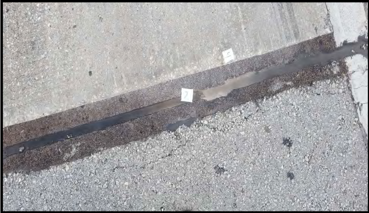
Photograph 9 View of Asbestos Homogeneous Area 3 – Closed-Cell Foam – Expansion Joint of Bridge 910001 (Sample Location 7).
