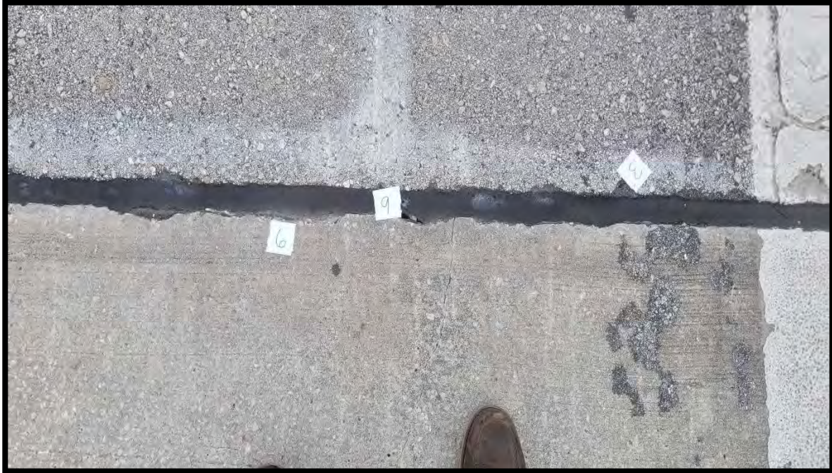
Photograph 11 View of Asbestos Homogeneous Area 3 – Closed-Cell Foam – Expansion Joint of Bridge 910001 (Sample Location 9).
