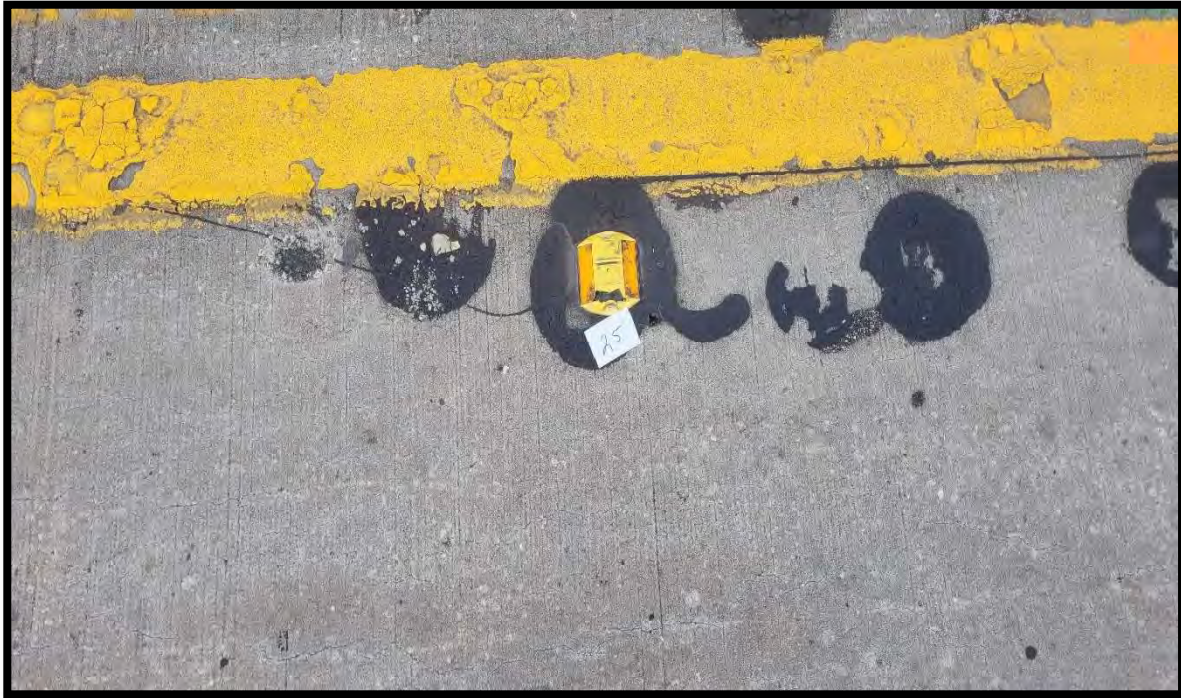
Photograph 27 View of Asbestos Homogeneous Area 9 – Black Adhesive – Surface Reflectors of Bridge 910001 (Sample Location 25).
