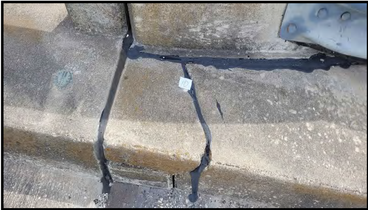
Photograph 12 View of Asbestos Homogeneous Area 4 – Bitumen Black Sealant – Seams and Cracks of Bridge 910001 (Sample Location 10).
