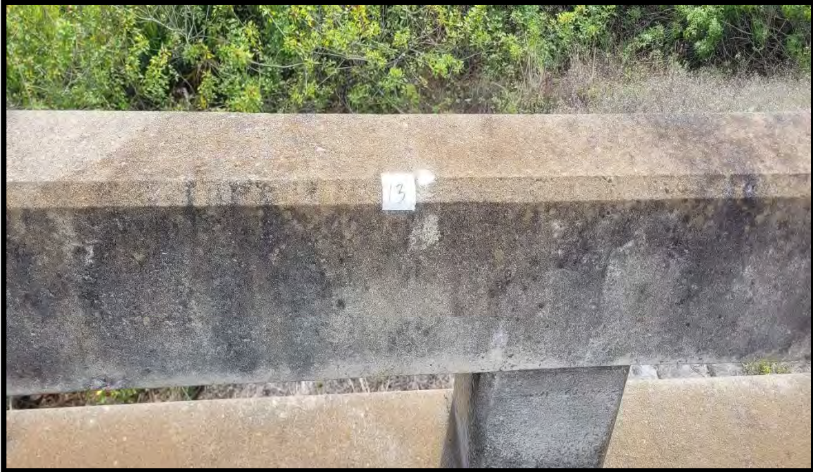
Photograph 15 View of Asbestos Homogeneous Area 5 – Concrete, Class V Coating – Guardrail of Bridge 910001 (Sample Location 13).
