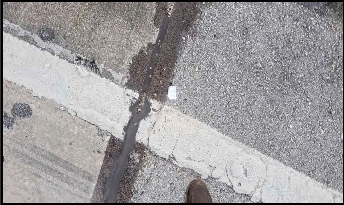
Photograph 3 View of Asbestos Homogeneous Area 1 – Asphalt – Approach Roadway of Bridge 910001 (Sample Location 1).
