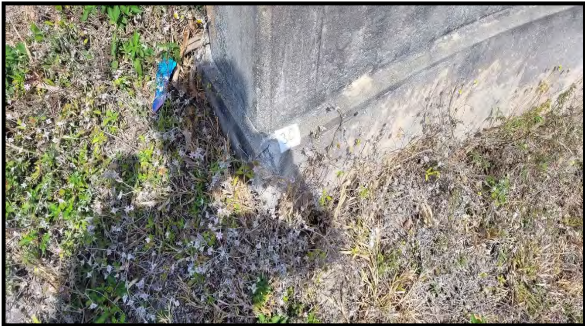
Photograph 32 View of Asbestos Homogeneous Area 10 – Concrete, Class V Coating – Landside Buttress of Bridge 910001 (Sample Location 30).
