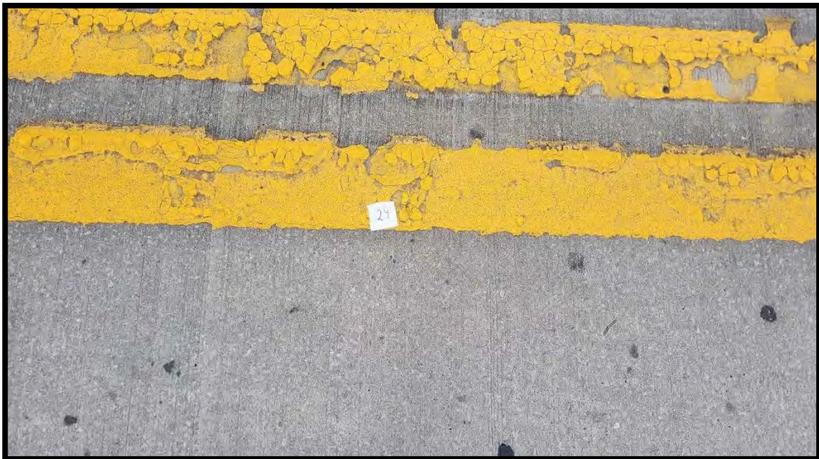
Photograph 26 View of Asbestos Homogeneous Area 8 – Yellow Lane Paint – Yellow Striping of Bridge 910001 (Sample Location 24).
