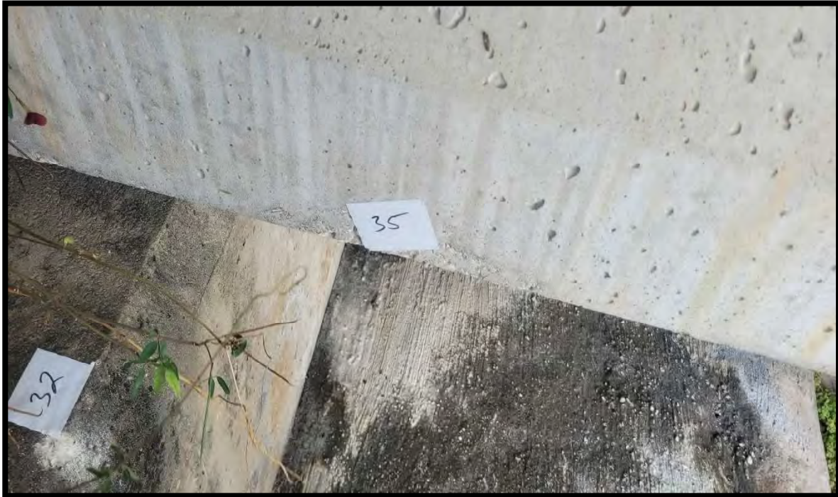
Photograph 37 View of Asbestos Homogeneous Area 12 – Concrete – Parallel I-Beam of Bridge 910001 (Sample Location 35).
