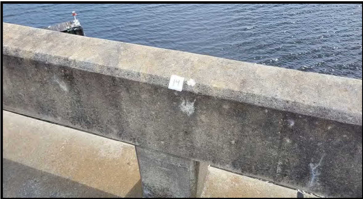
Photograph 16 View of Asbestos Homogeneous Area 5 – Concrete, Class V Coating – Guardrail of Bridge 910001 (Sample Location 14).
