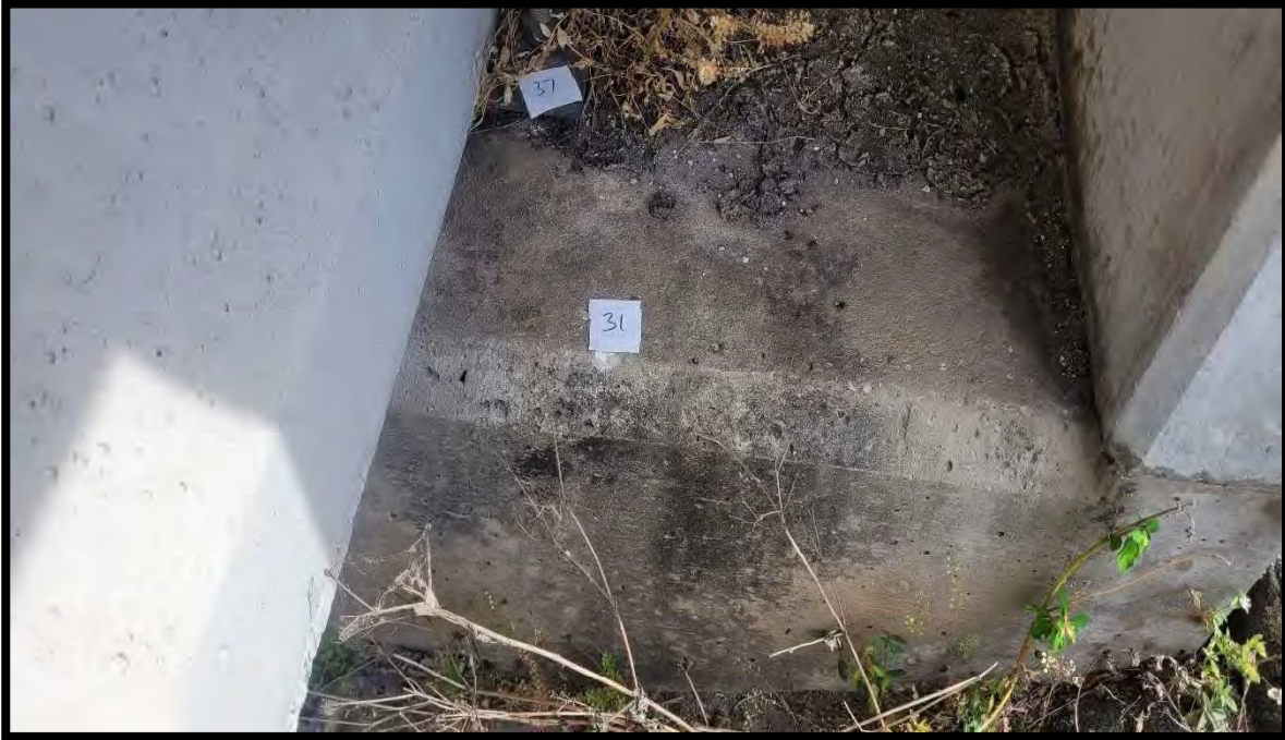
Photograph 33 View of Asbestos Homogeneous Area 11 – Concrete – Pylon Cap (Perpendicular Beam) of Bridge 910001 (Sample Location 31).
