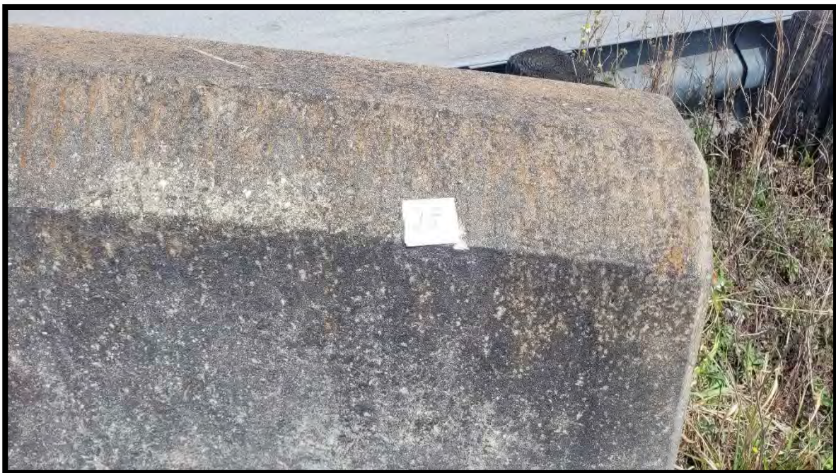
Photograph 30 View of Asbestos Homogeneous Area 10 – Concrete, Class V Coating – Landside Buttress of Bridge 910001 (Sample Location 28).
