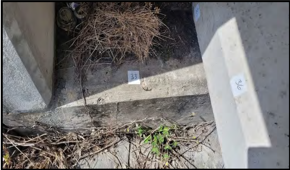
Photograph 35 View of Asbestos Homogeneous Area 11 – Concrete – Pylon Cap (Perpendicular Beam) of Bridge 910001 (Sample Location 33).
