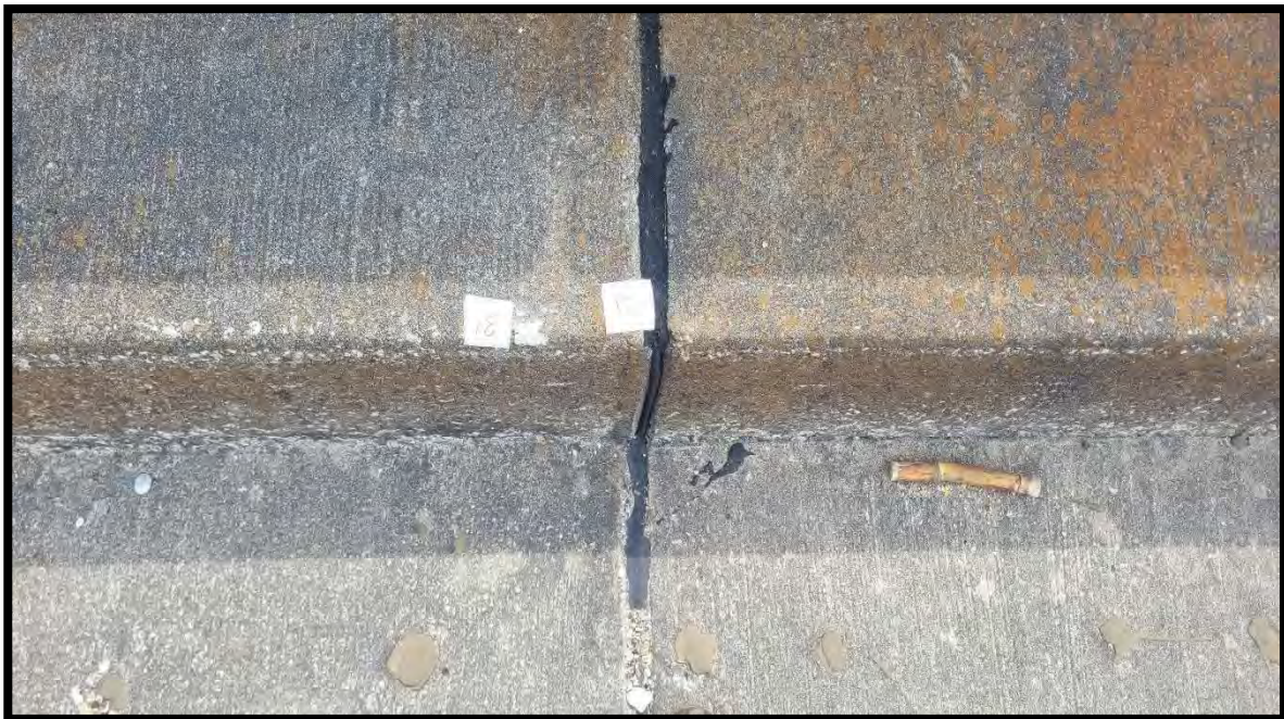
Photograph 14 View of Asbestos Homogeneous Area 4 – Bitumen Black Sealant – Seams and Cracks of Bridge 910001 (Sample Location 12).
