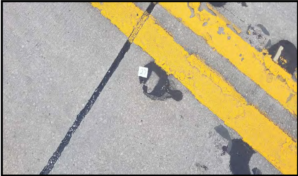
Photograph 29 View of Asbestos Homogeneous Area 9 – Black Adhesive – Surface Reflectors of Bridge 910001 (Sample Location 27).
