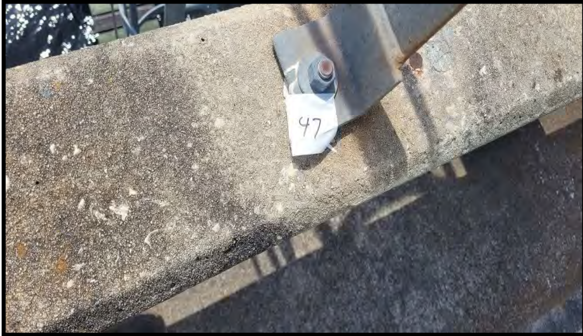
Photograph 49 View of Asbestos Homogeneous Area 16 – White Caulk – Ladder Anchor Points of Bridge 910001 (Sample Location 47).
