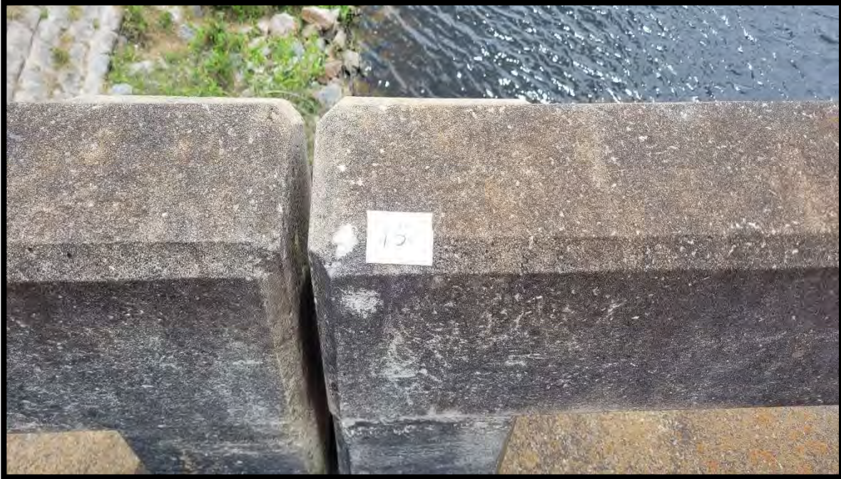
Photograph 17 View of Asbestos Homogeneous Area 5 – Concrete, Class V Coating – Guardrail of Bridge 910001 (Sample Location 15).
