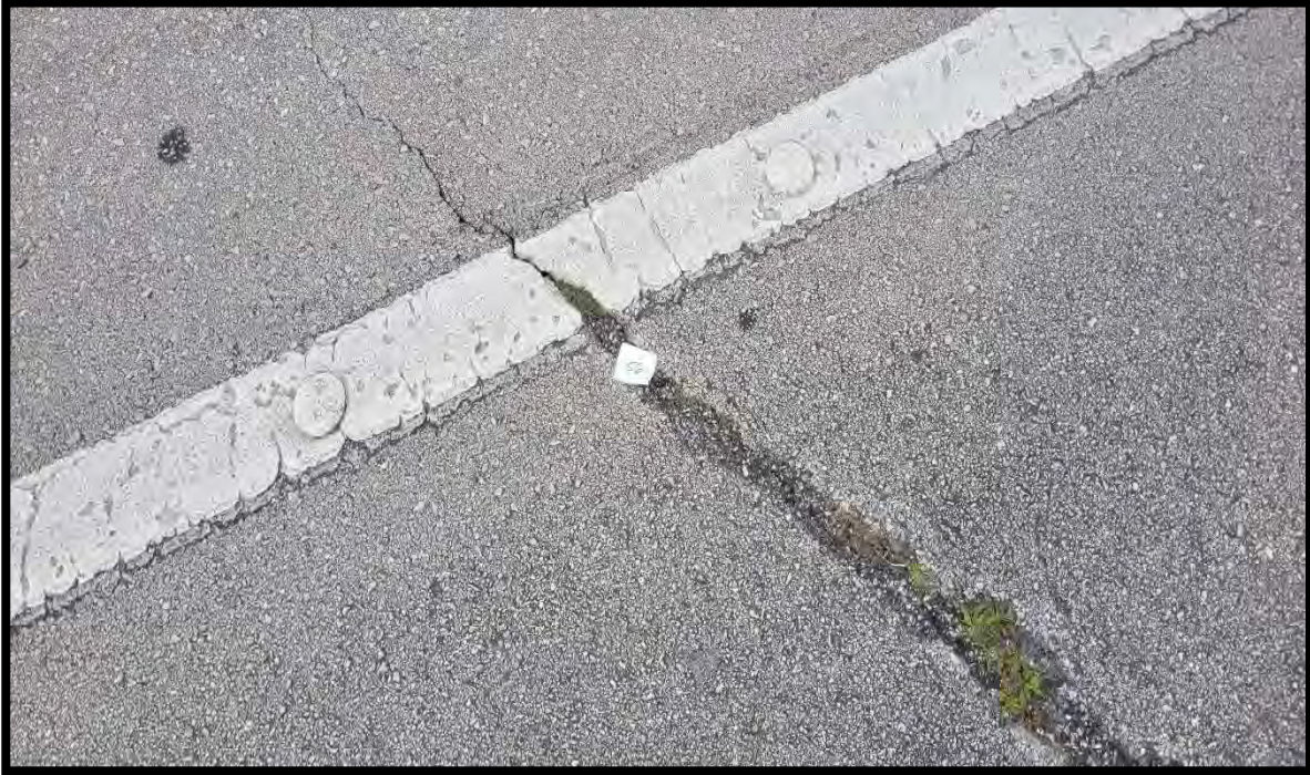
Photograph 57 View of Asbestos Homogeneous Area 19 – Asphalt – Expansion Joint of Bridge 910002 (Sample Location 56).
