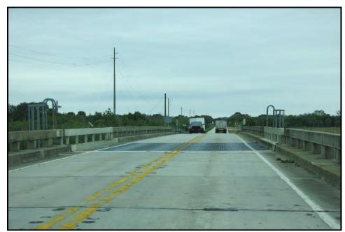
**Photo 5.10.** SR 70 over Kissimmee River Bridge (FDOT 910001) (8HG01236/8OB00336), looking east. Note the removable steel span.
