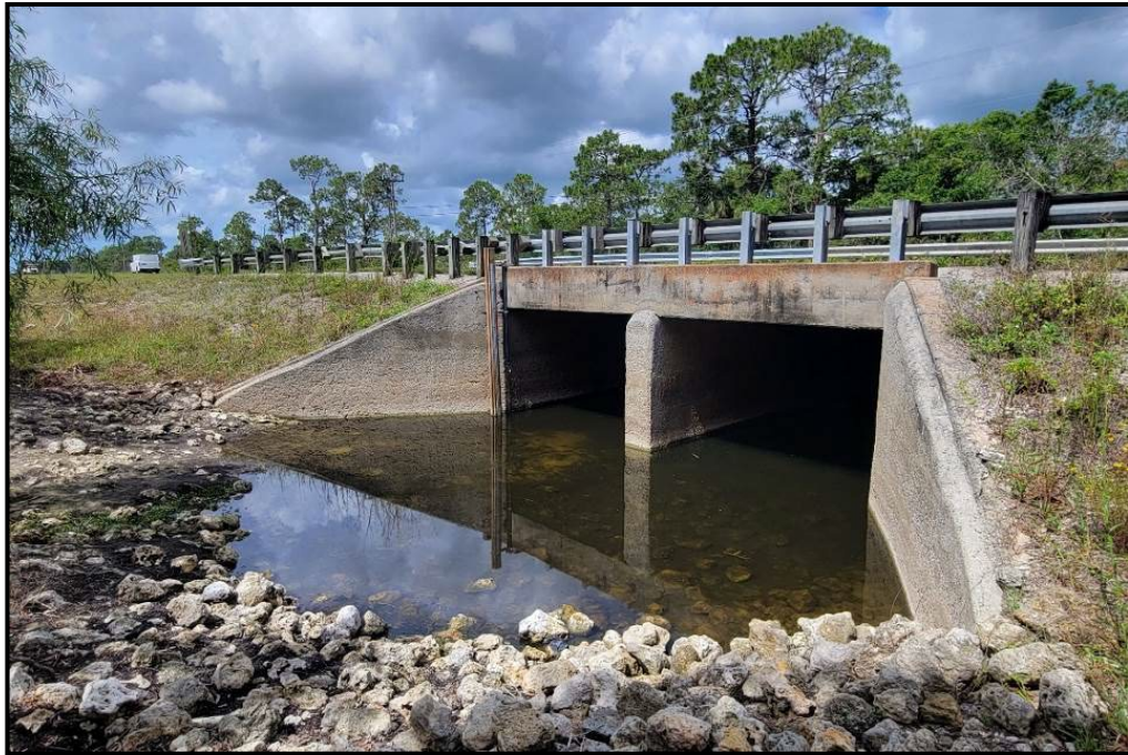
Photo 5.6. Burnt Store Road over Yucca Pen Creek (FDOT Bridge No. 120024) (8LL02875), a concrete box culvert, looking southwest.
