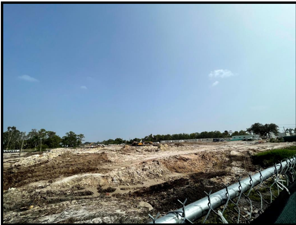
Photos: Area Under Construction
