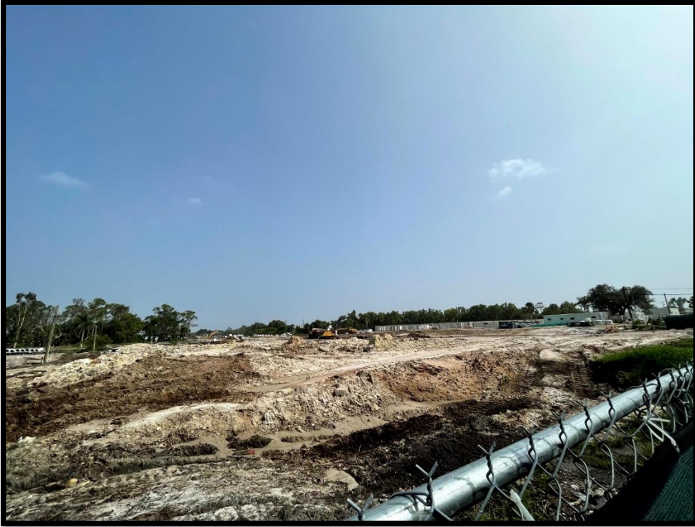
Photo 5: Area under construction adjacent to project limits
