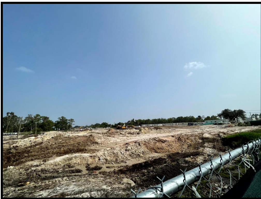
Photos: Area Under Construction
