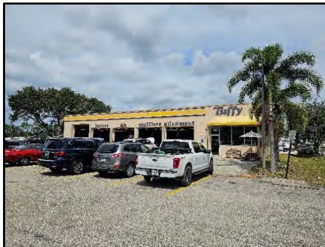
Photo 2.10. Building conditions within Pond West facing northwest.
